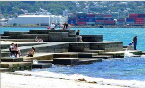
Terraced seawalls absorb and dissipate wake energy and allow people to touch the water
