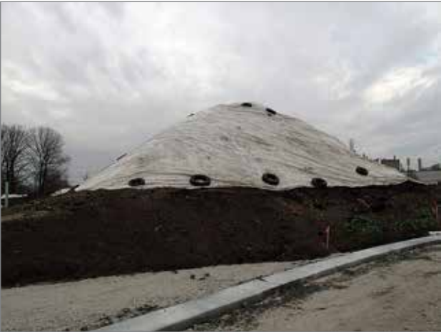
Stockpile topsoil on site to prevent its loss on-site
