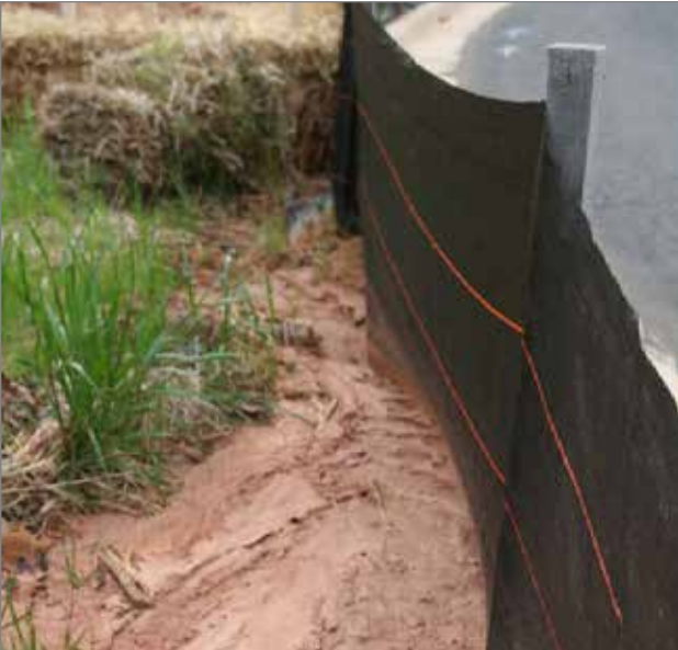
Sediment traps and silt fencing can help prevent the sedimentation of storm sewers and receiving streams
